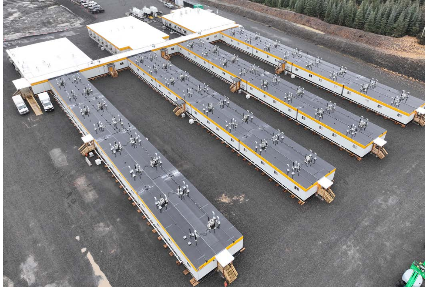
CAMP 11 WORK AREA
