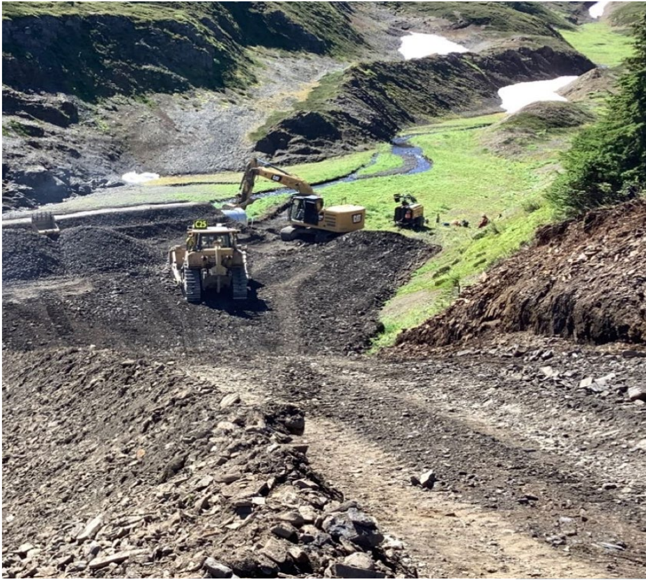
Coulter Creek Access Road
