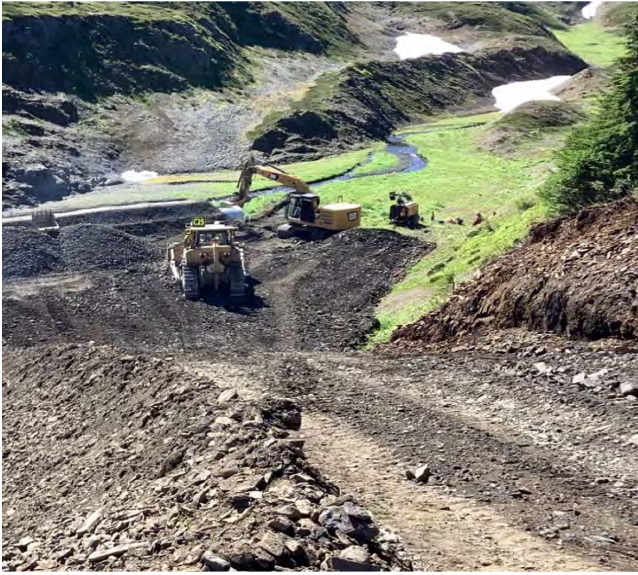
Coulter Creek Access Road
