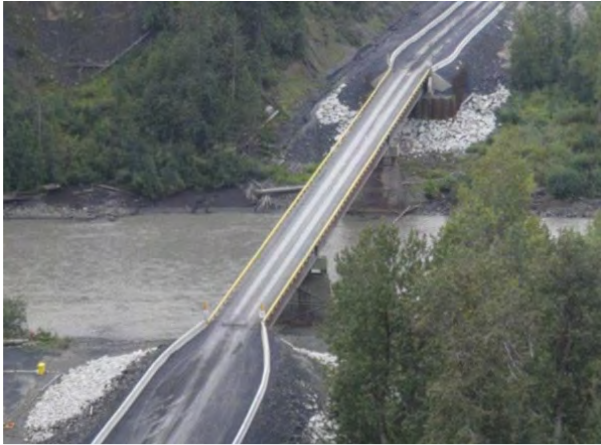
Bell-Irving Bridge completed
