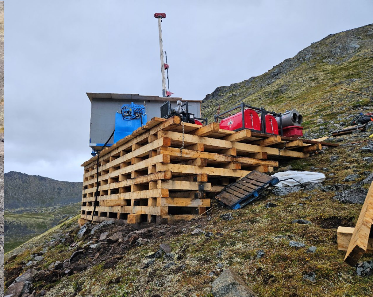
Drill on Deck and drilling away end of August 2023
