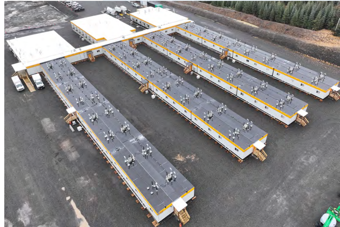
CAMP 11 WORK AREA
