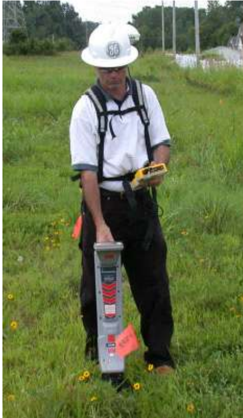
Figure 1: Locating the centreline a pipe locator.
