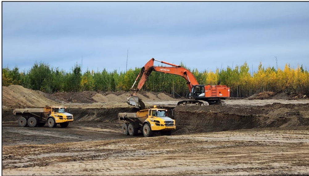
Extracting Material from Borrow Source along New Mine Access Road
