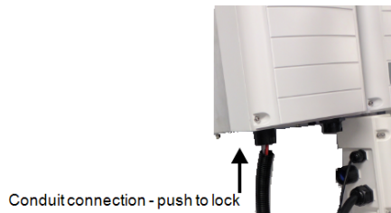
Figure 25: Connecting the conduit to the Secondary Unit
