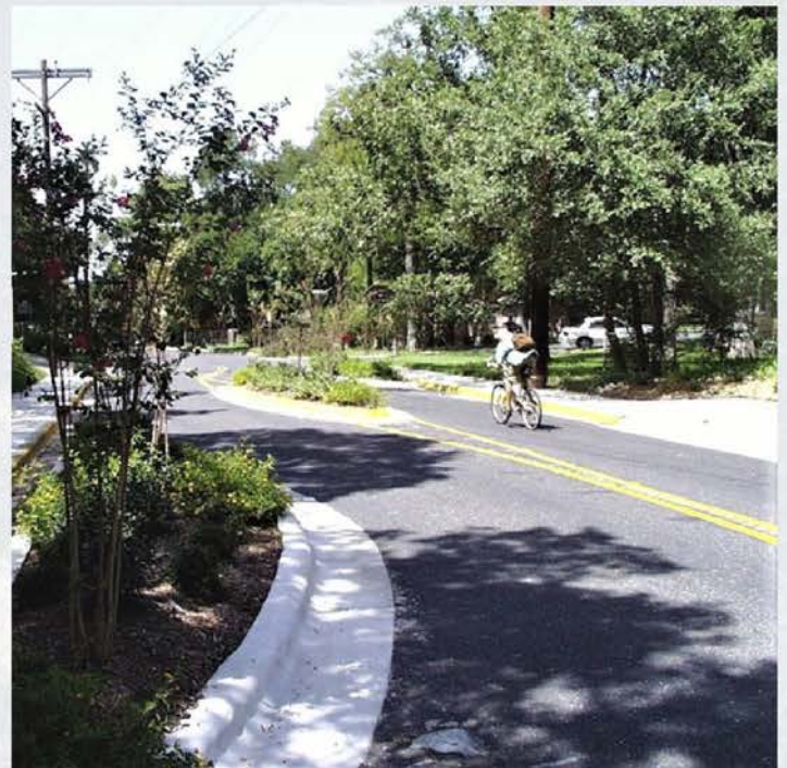
OFFSET CURB EXTENSION, ALSO CALLED CHICANES, CAN SLOW TRAFFIC SPEEDS
