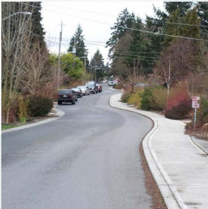
OFFSET CURB EXTENSION, ALSO CALLED CHICANES, CAN SLOW TRAFFIC SPEEDS
