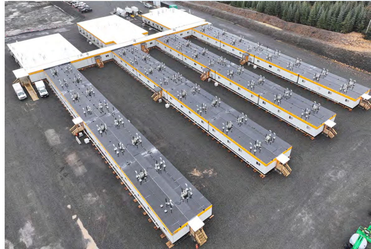
CAMP 11 WORK AREA
