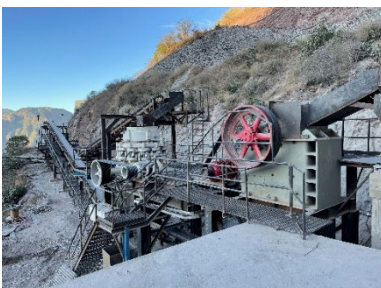
New Permanent Crushing Circuit
