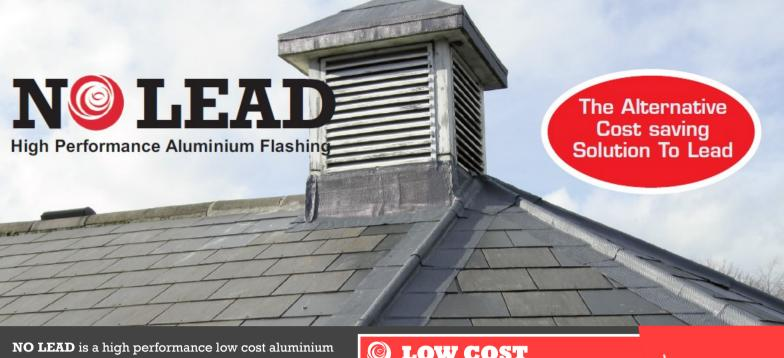
flashing suitable for use as an alternative to traditional lead in both flat and pitched roof applications.
