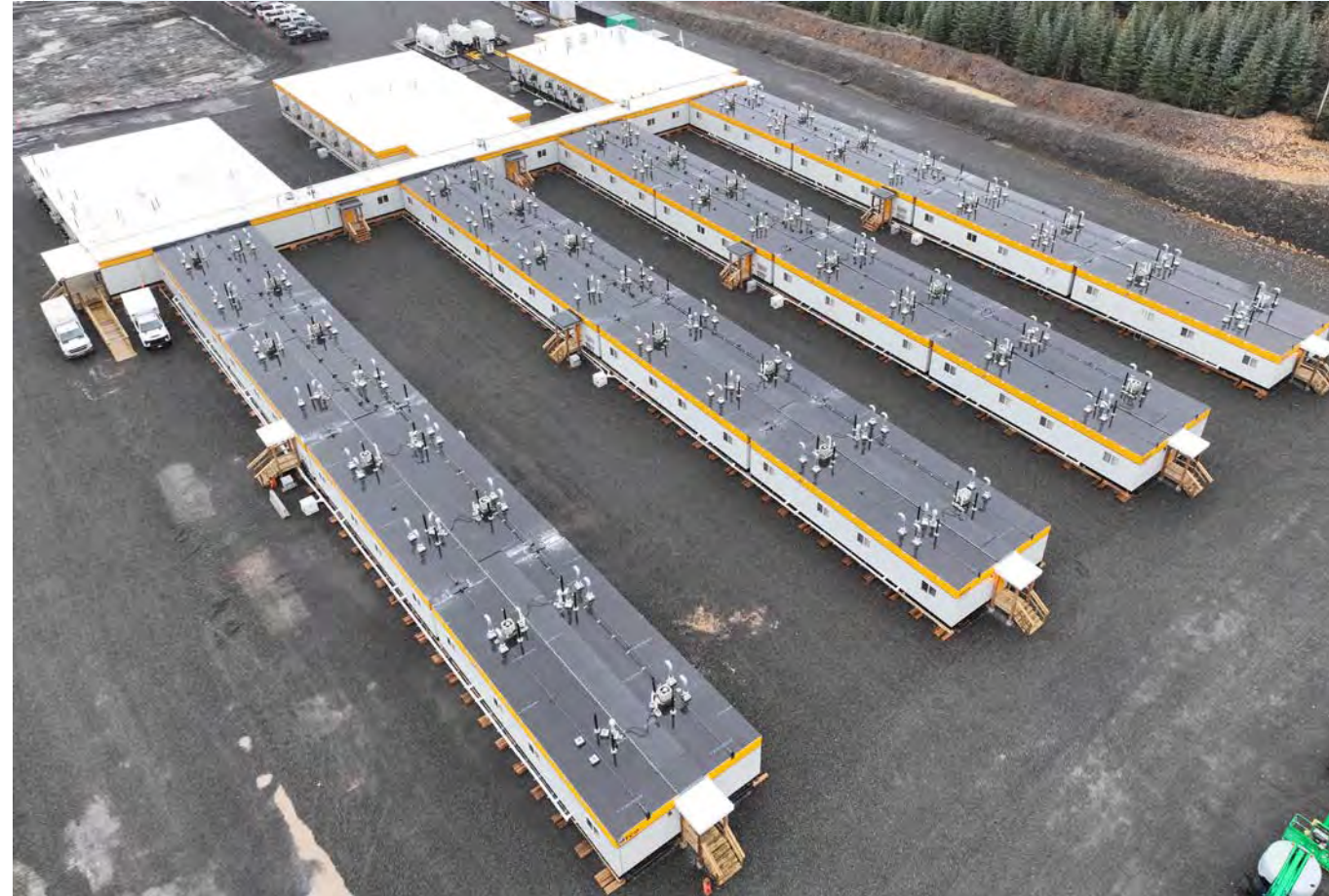
CAMP 11 WORK AREA
