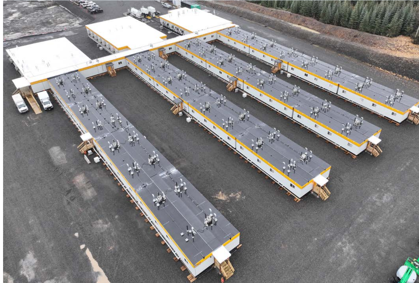
CAMP 11 WORK AREA
