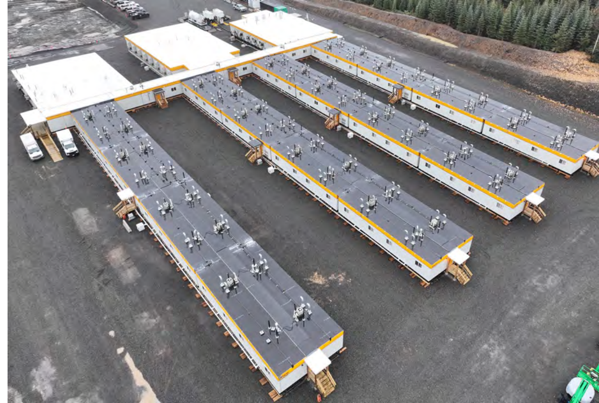
CAMP 11 WORK AREA
