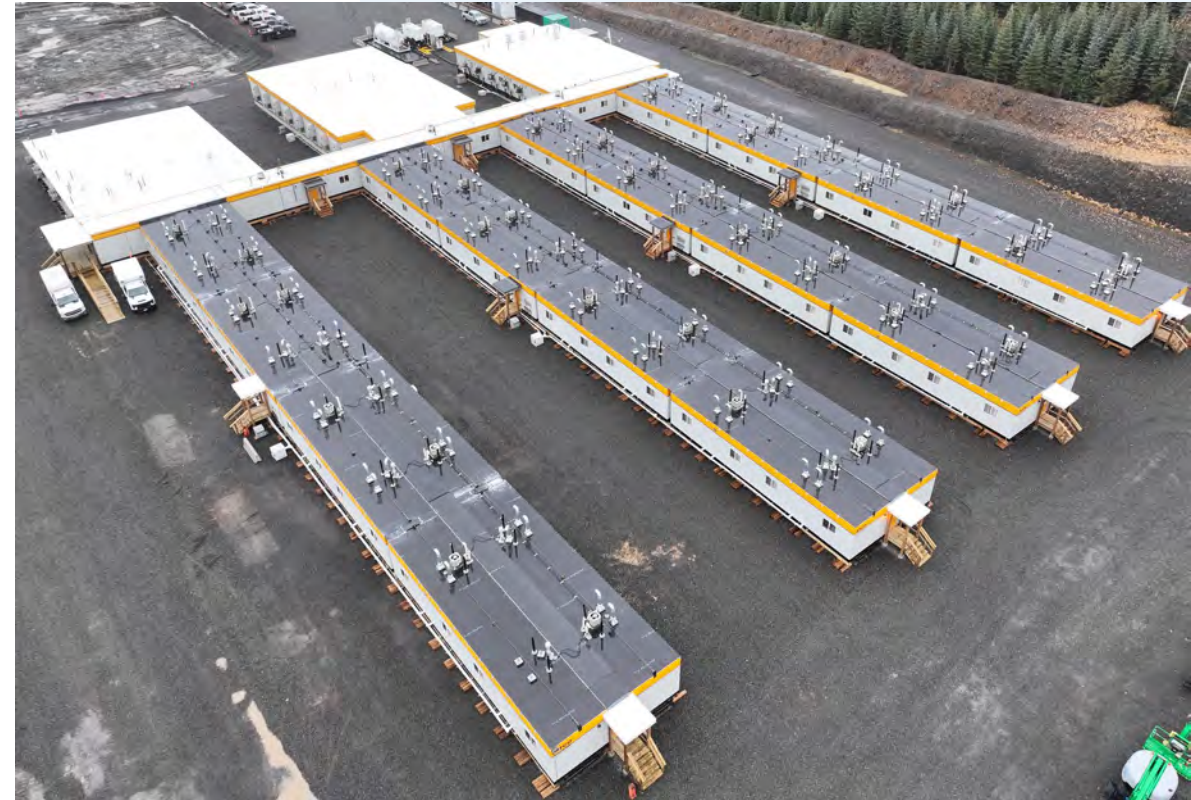
CAMP 11 WORK AREA
