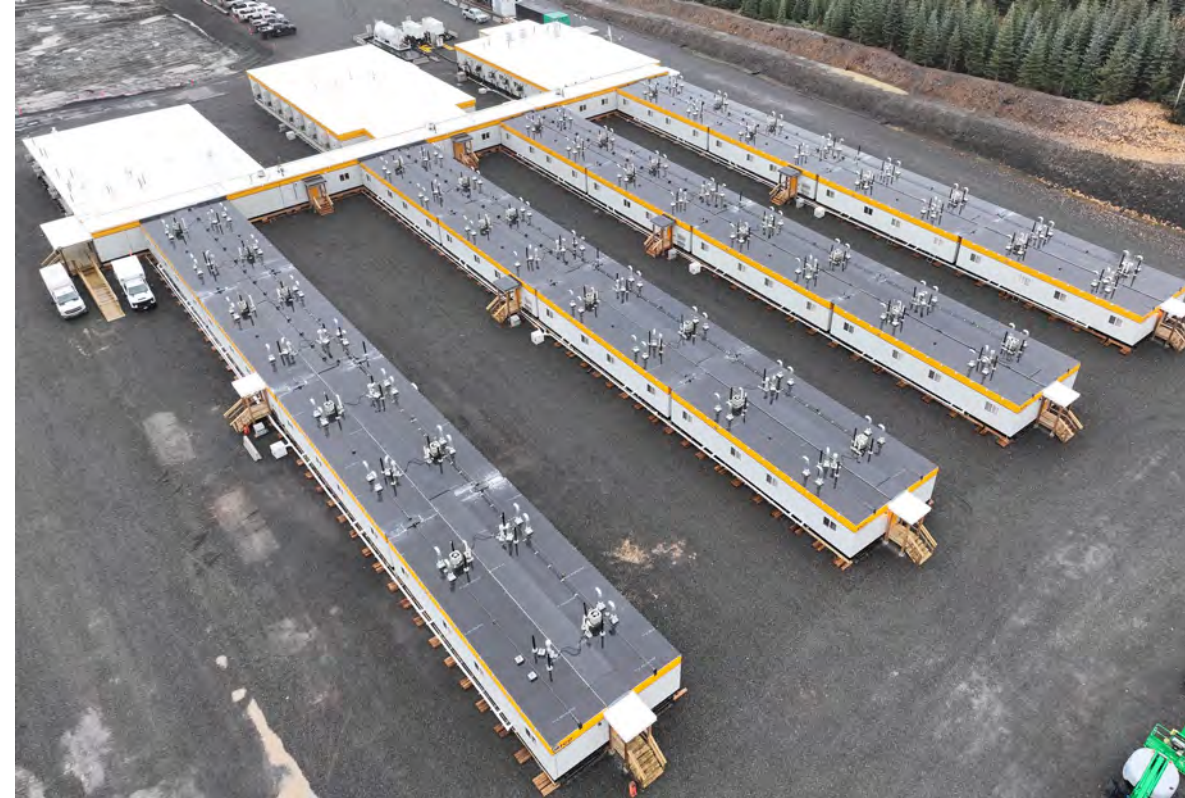
CAMP 11 WORK AREA
