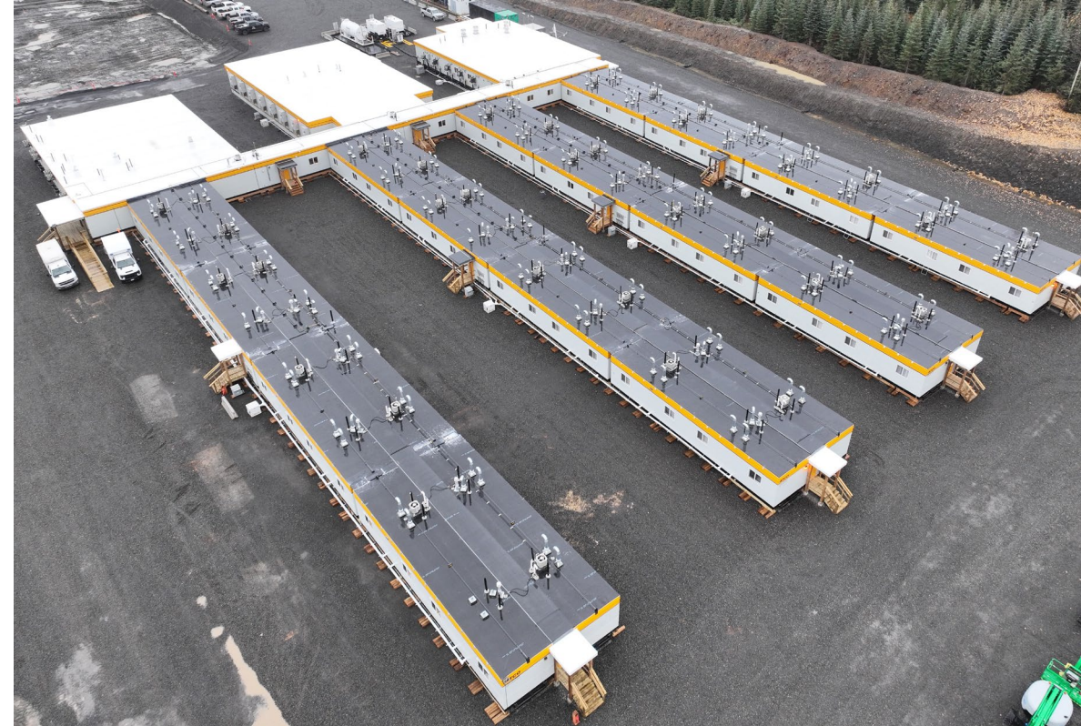
CAMP 11 WORK AREA
