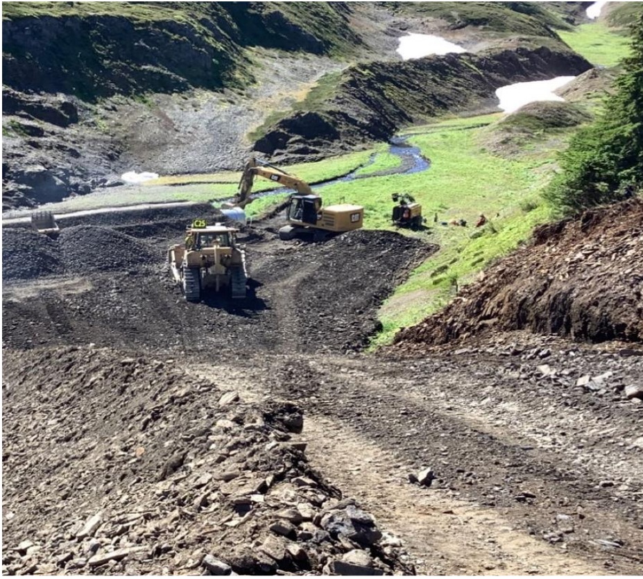
Coulter Creek Access Road
