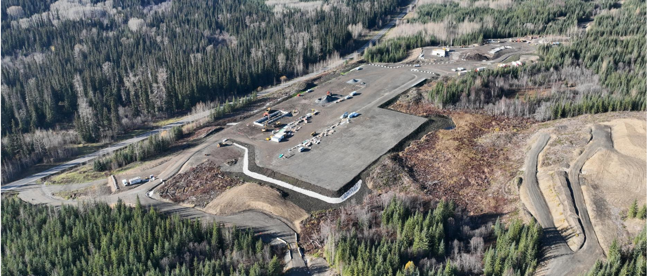
BC Hydro's Treaty Creek Terminal
