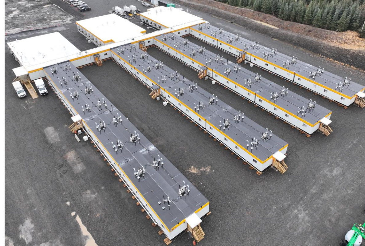
CAMP 11 WORK AREA
