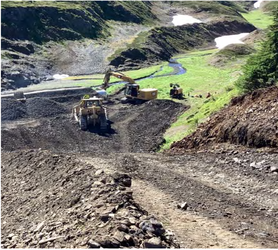
Coulter Creek Access Road
