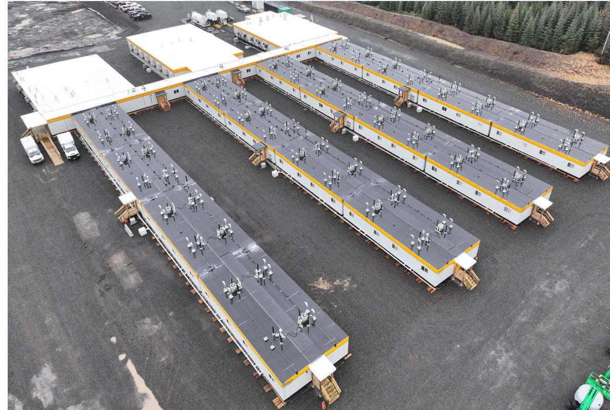
CAMP 11 WORK AREA
