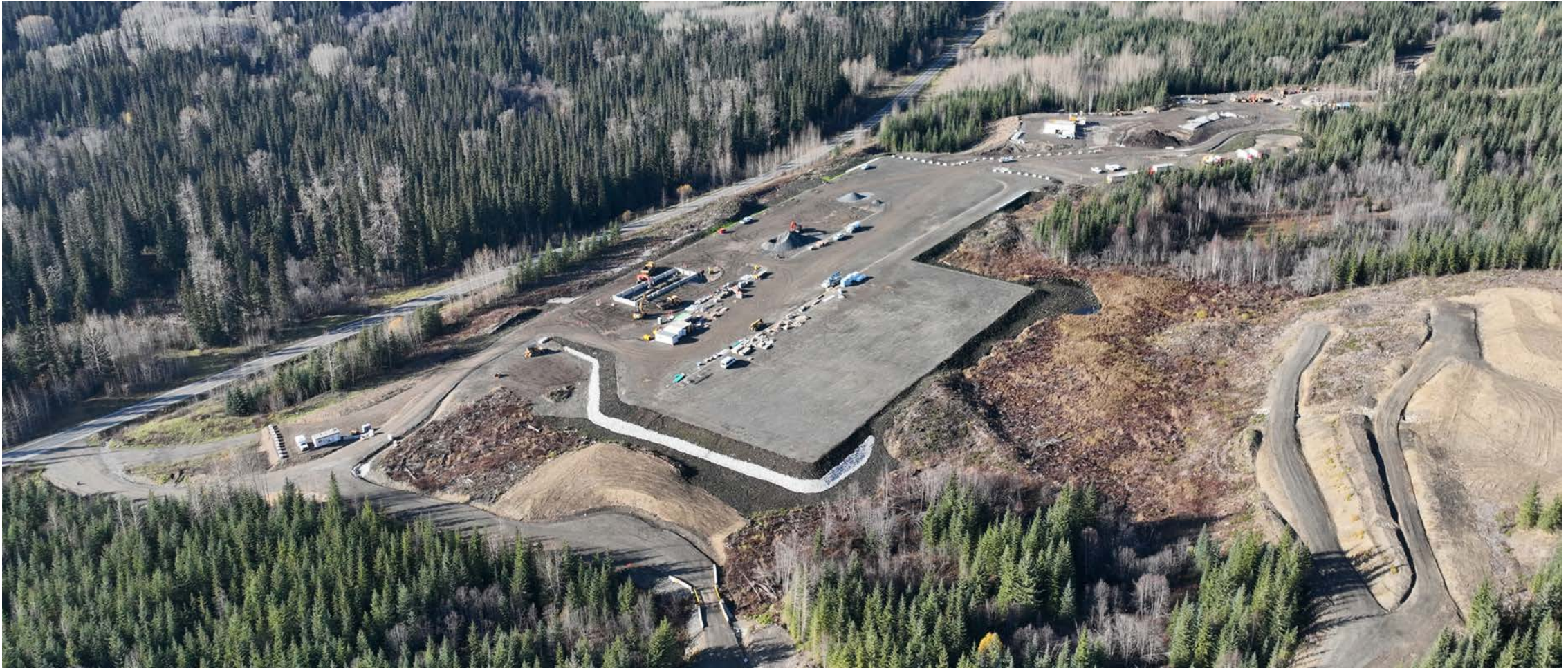
BC Hydro's Treaty Creek Terminal
