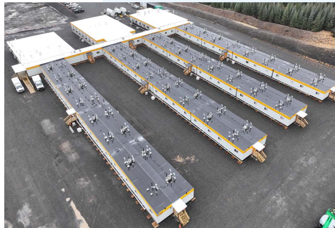
CAMP 11 WORK AREA
