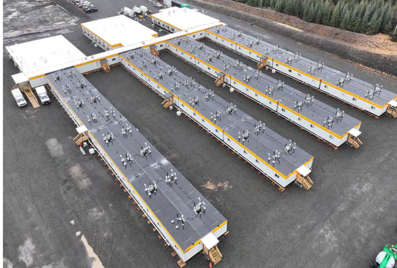
CAMP 11 WORK AREA
