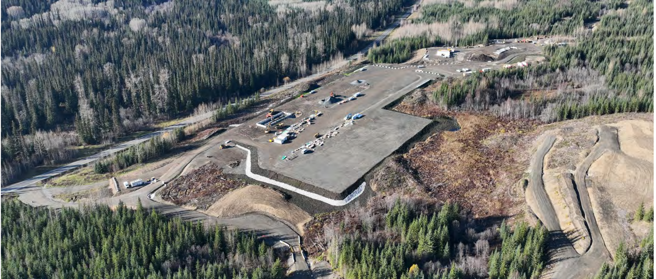
BC Hydro's Treaty Creek Terminal
