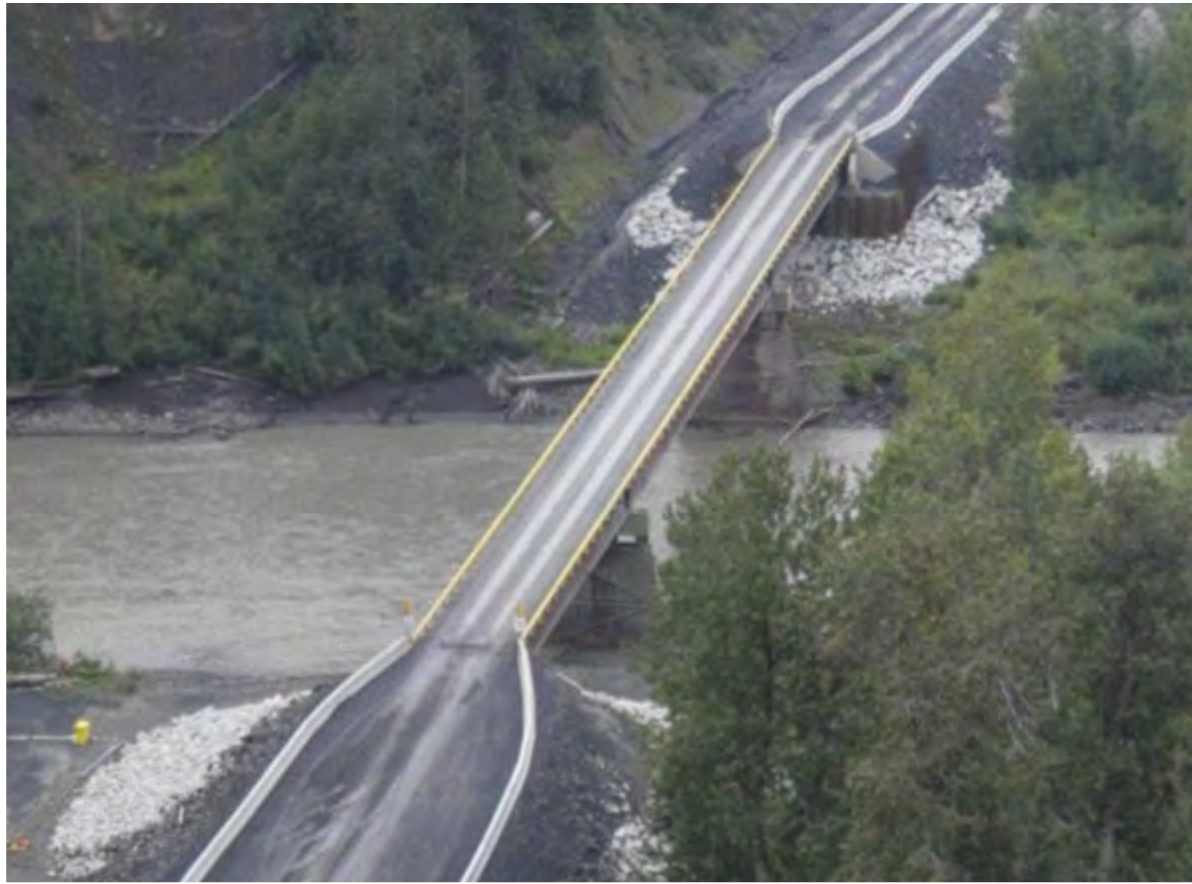
Bell-Irving Bridge completed
