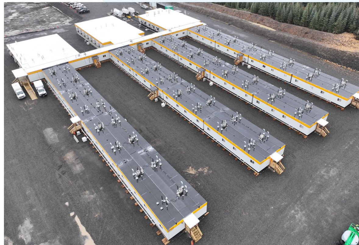
CAMP 11 WORK AREA
