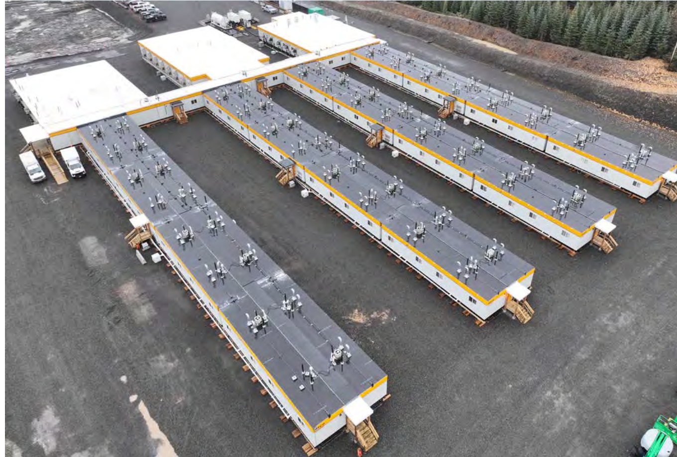
CAMP 11 WORK AREA
