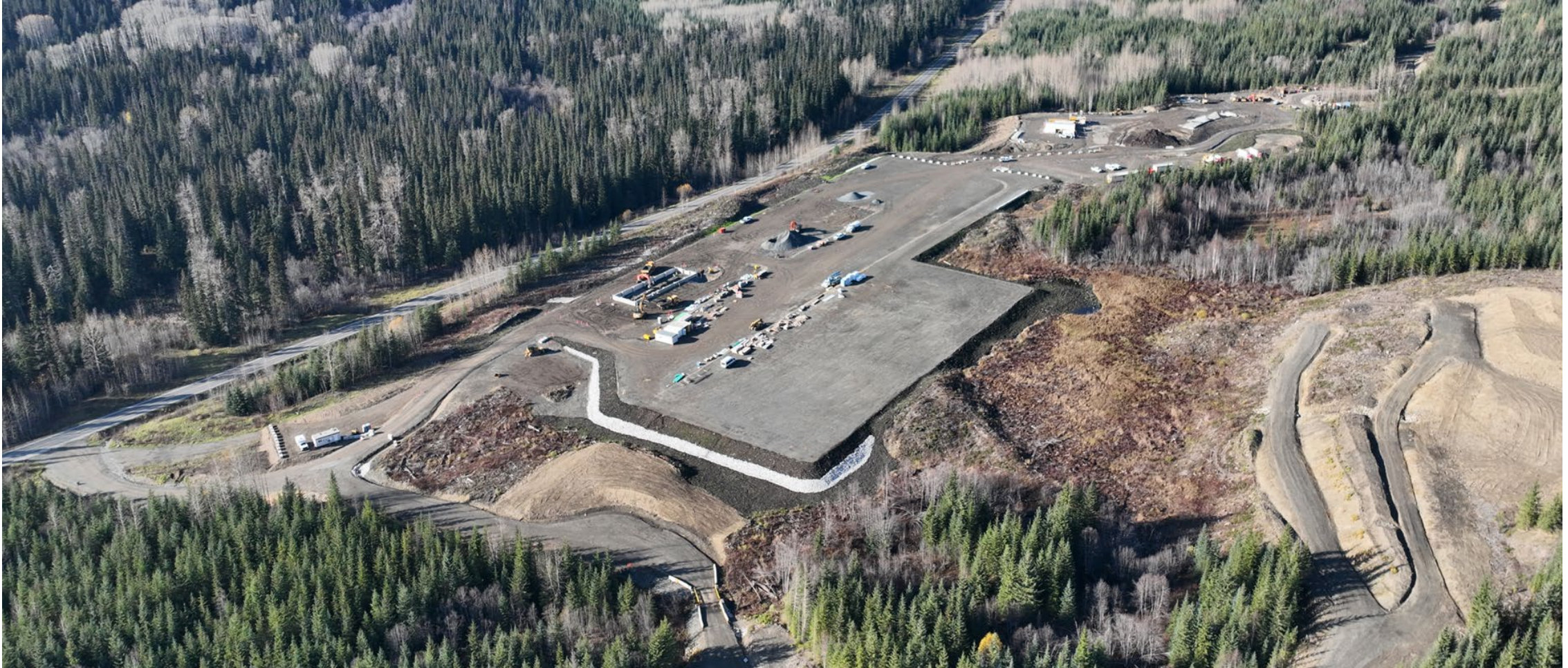
BC Hydro's Treaty Creek Terminal
