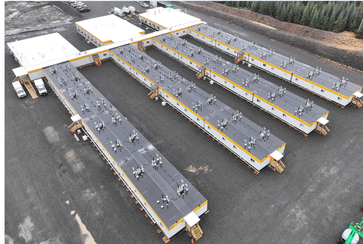
CAMP 11 WORK AREA
