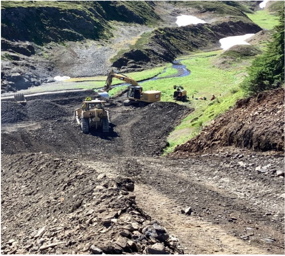
Coulter Creek Access Road
