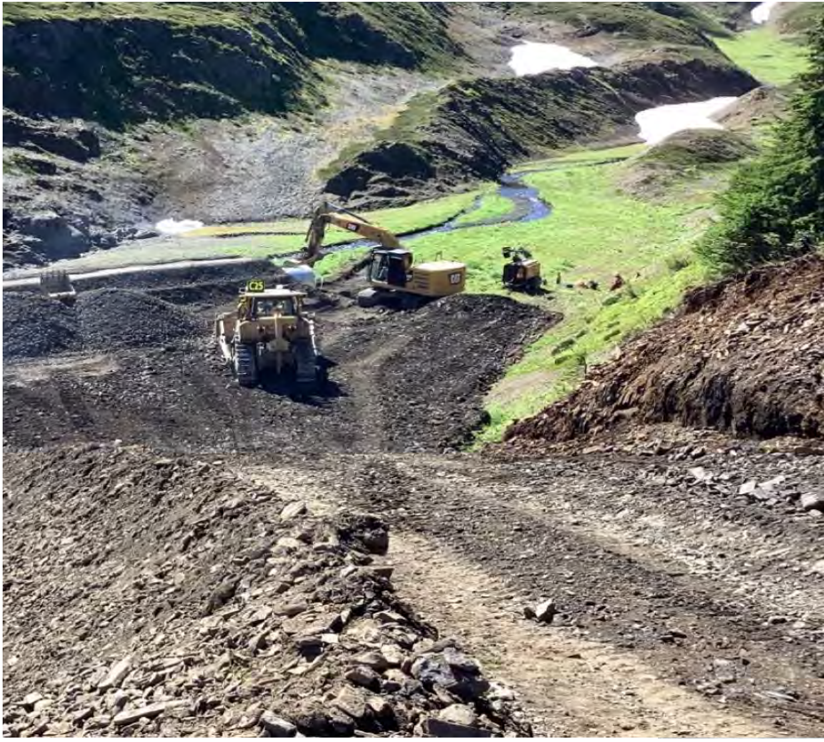
Coulter Creek Access Road
