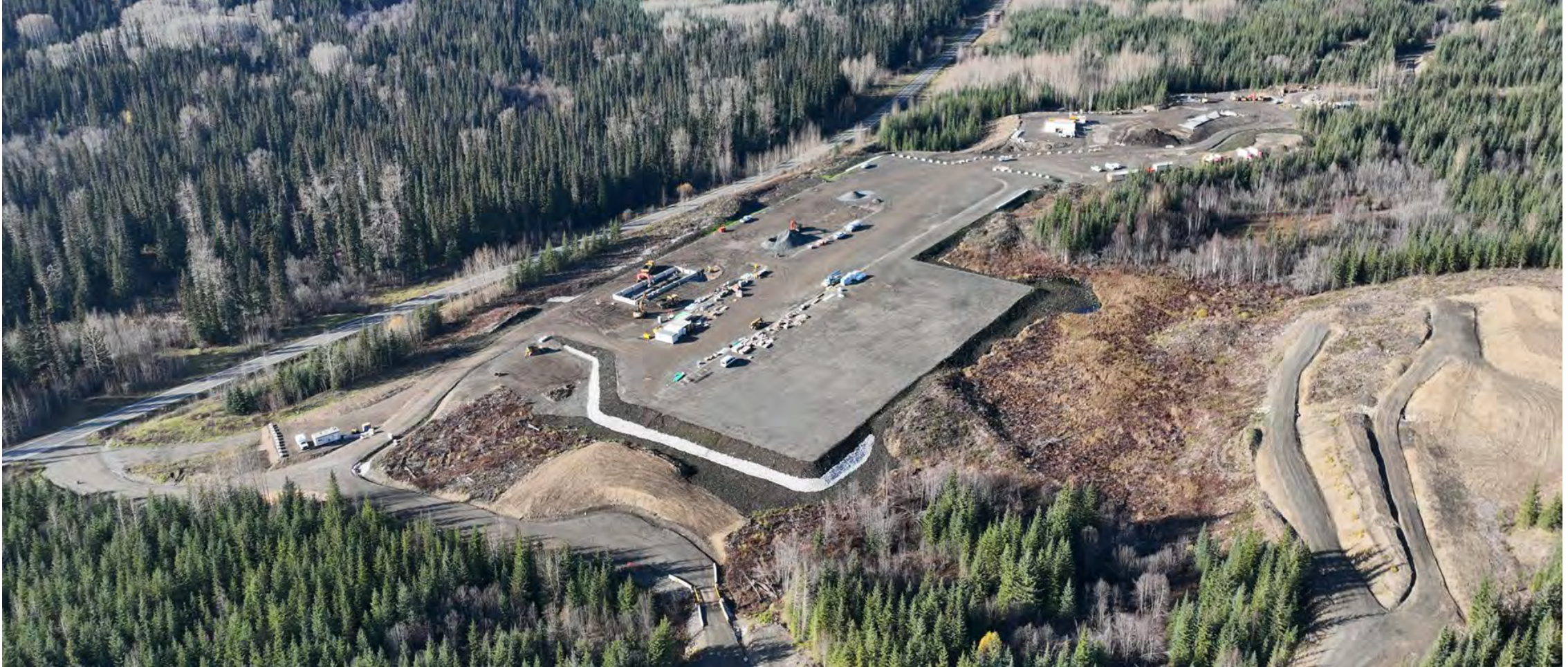
BC Hydro's Treaty Creek Terminal
