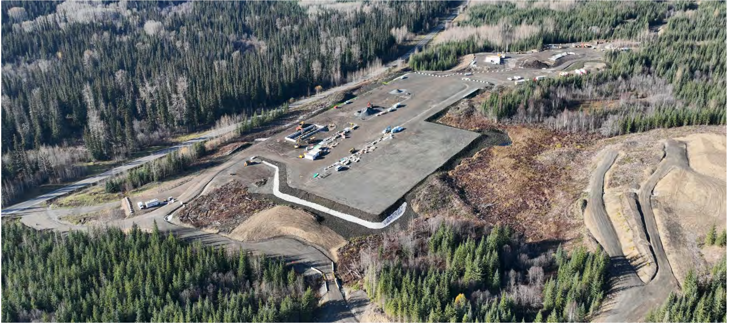
BC Hydro's Treaty Creek Terminal
