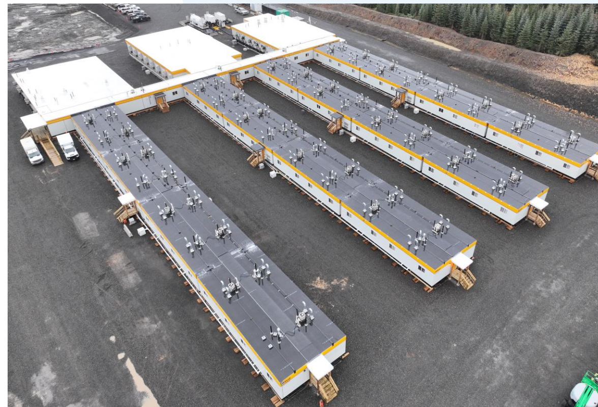
CAMP 11 WORK AREA
