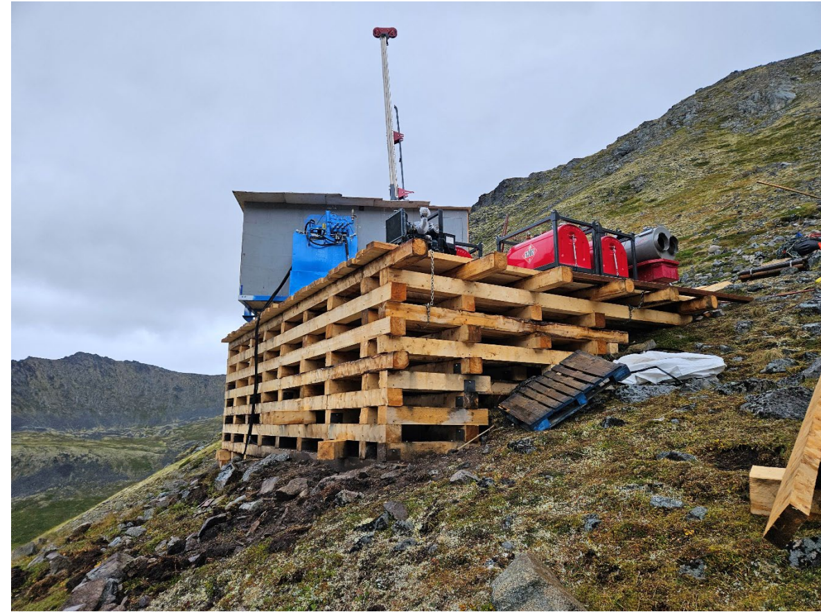
Drill on Deck and drilling away end of August
